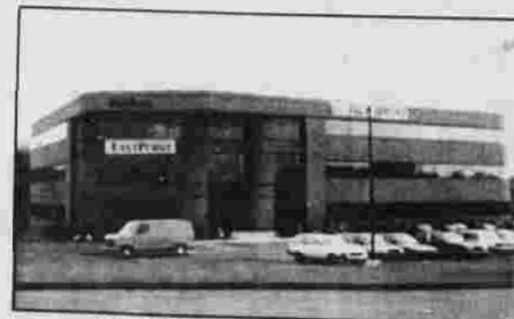
EAST POINT BUSINESS CENTER
